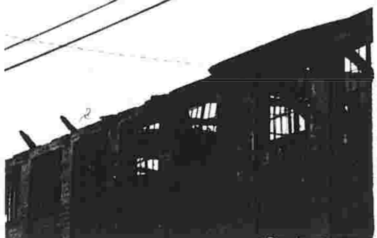
OLD BON AMI PLANT HILLIARD STREET
